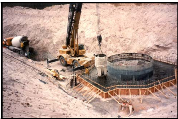
Shaft frame construction
