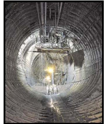
Completed inset with steel rings and concrete backfilling
