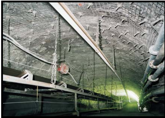
Tunnel Lining and Bolting Techniques
