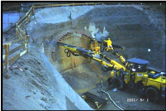
Gräbern Tunnel - tube umbrella
