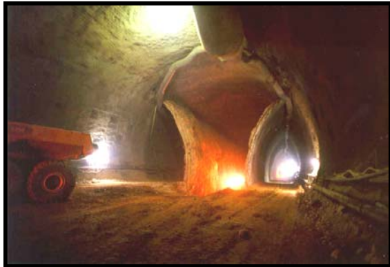
Dembach road tunnel - Germany
