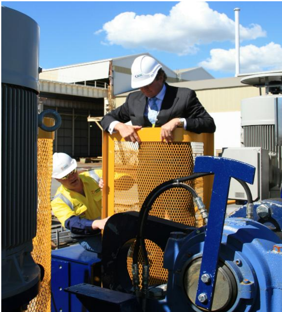
Andrew Forrest getting shown the workings of the Train Unloader Indexer by Marc Humm (TUL Project Manager – Metso AP).
