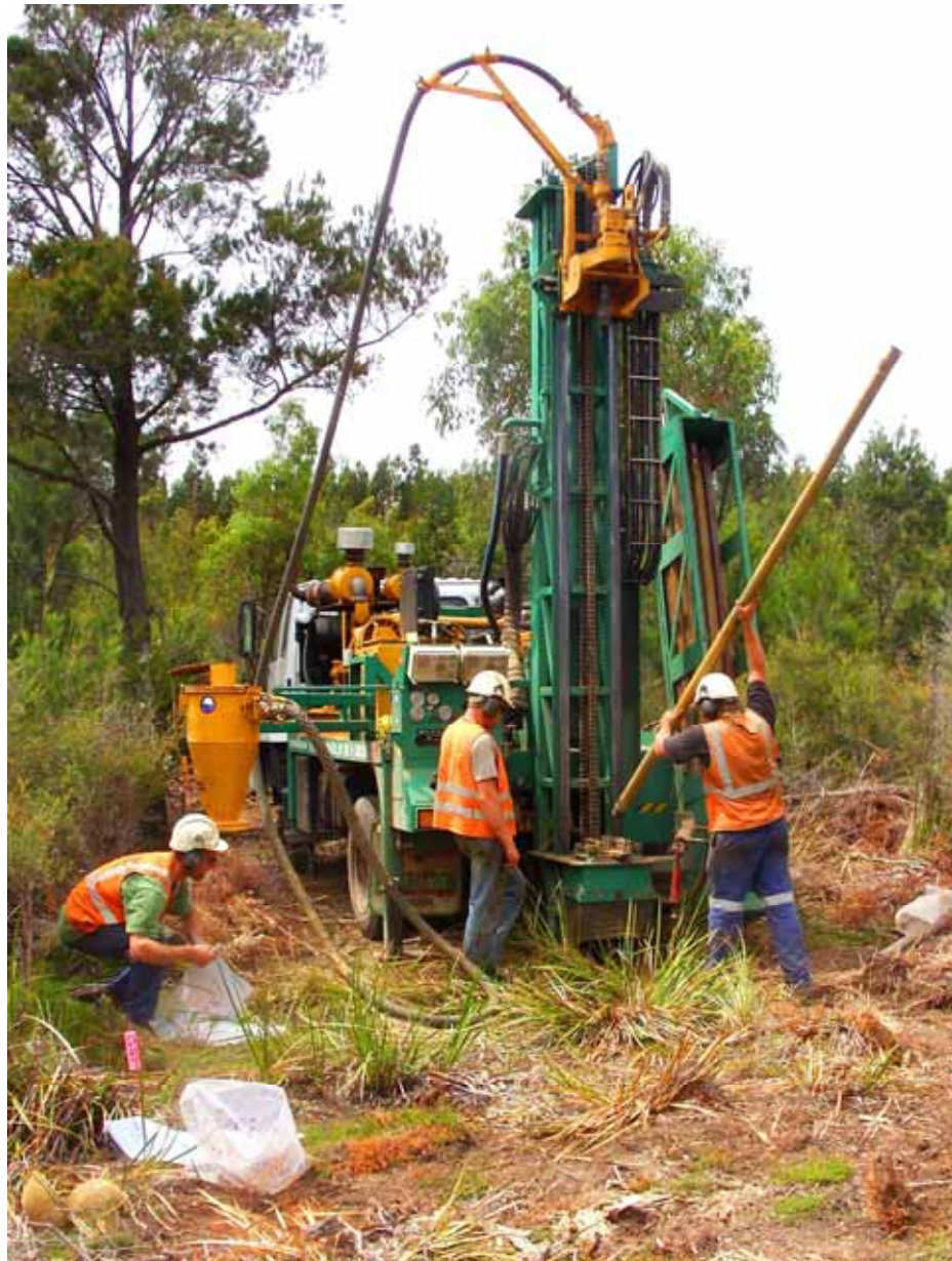
Figure 3 – Aircore Drilling at Barnes Hill
