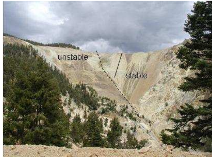
Figure 8: Goathill North rock pile before re-grading and looking east. Solid line indicates approximate location of trenches completed in summer-fall 2004; dashed line indicates the boundary between the stable and unstable portions of the rock pile (after McLemore et al., 2006)
