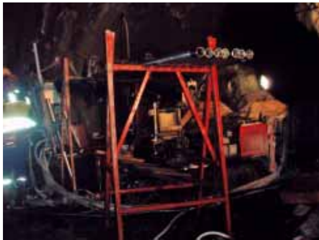
Diamond drilling contractor Drillcon SMOY operating a new Sandvik core drill, mounted on a mini-excavator crawler chassis, underground at Pampalo
