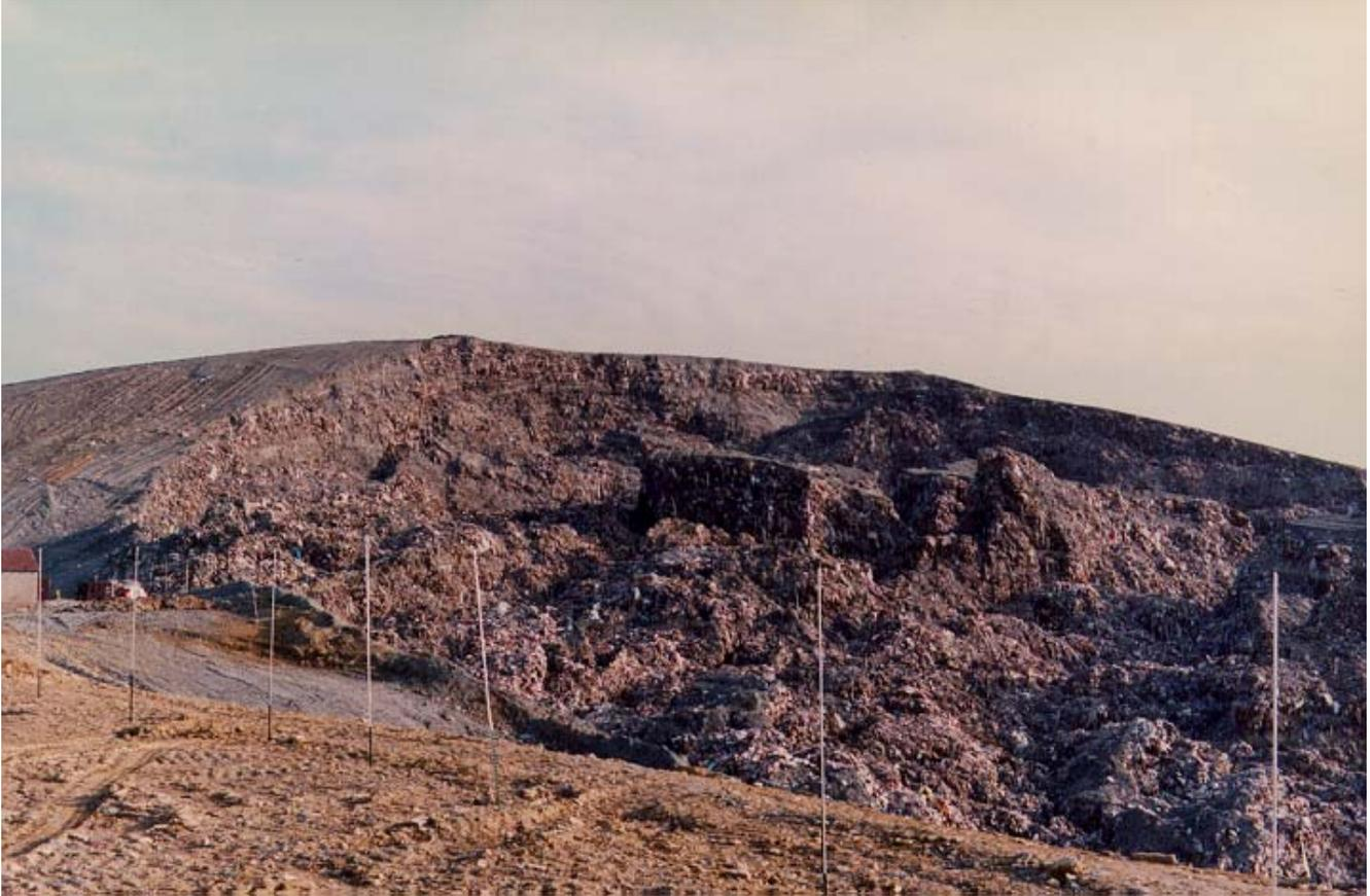
Figure 9. MSW Slope Failure at the Rumpke Landfill
