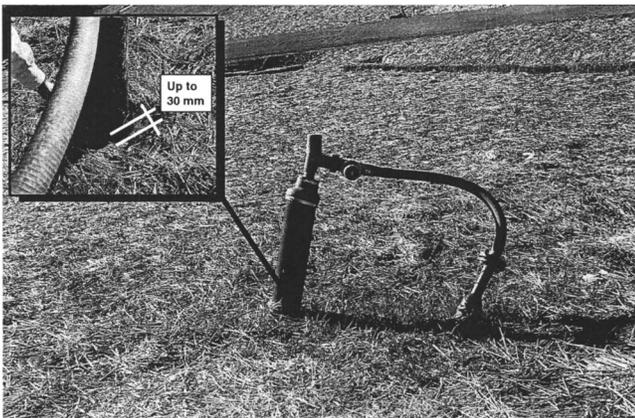
**Fig. 4.** Landfill gas riser displaced by cover soil movement
