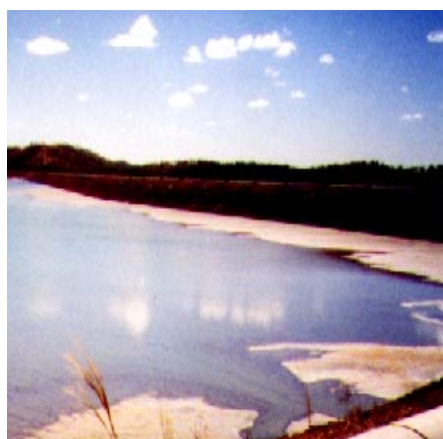
Beaching against walls may allow granivorous birds to access tailing liquor.
