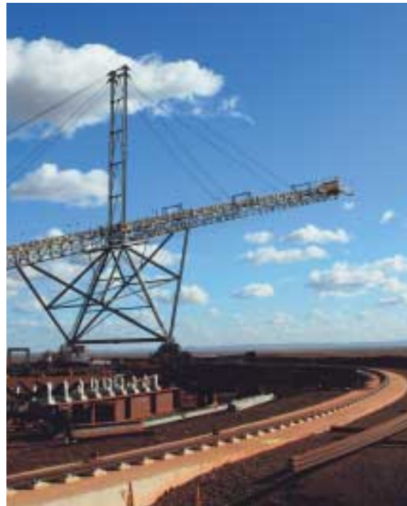
Stacker mounted on ring-beam at Cloud Break
