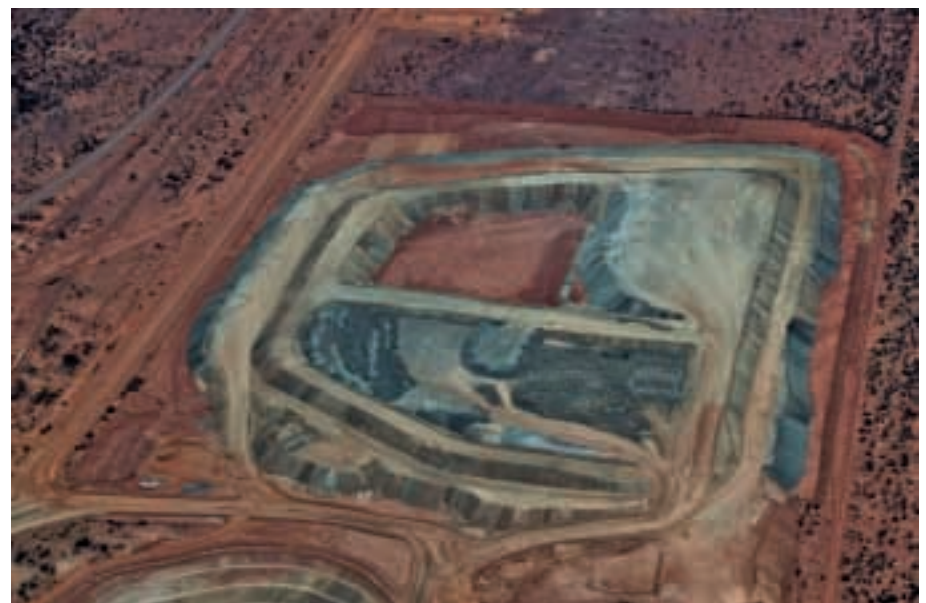
Same dump as above during construction. Different material types identifiable
