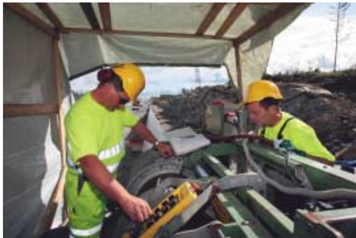
Installing KWH pipe at Talvivaara (Photo by Arto Tulima)
