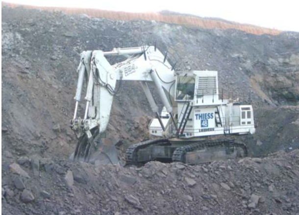
Photo 3 Excavator at Collinsville with guidance used to find the edge of Coal.
