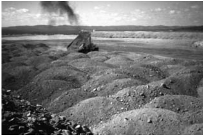
Figure 2. Placement of rocky soil mulch layer on South Pile cover trial.
