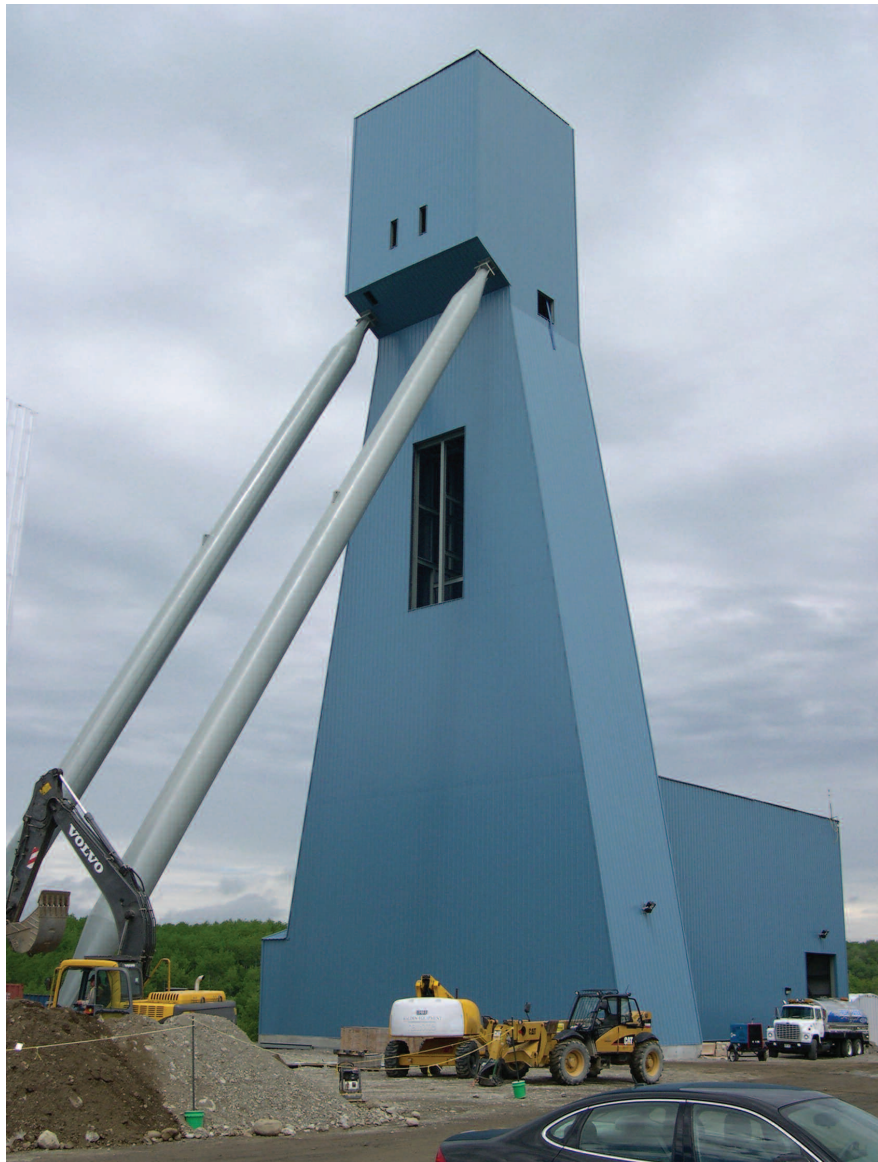
Vale Inco Totten mine headframe under construction - June 2008
