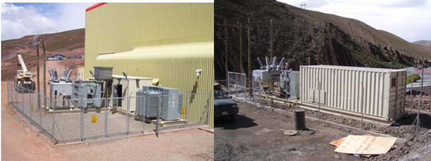
SKID MOUNTED SUBSTATIONS
